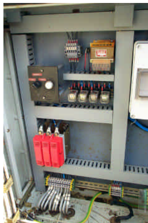
heating switcher cabinet
