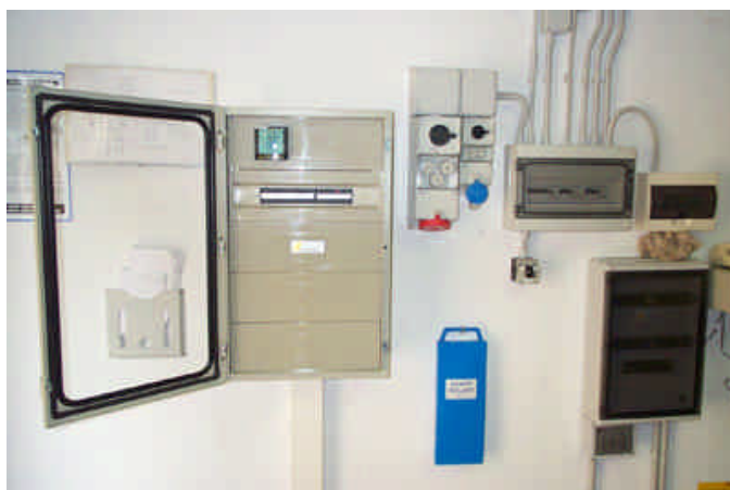
Control unit installation
