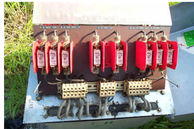
380V/55V Transformer (resistor)
