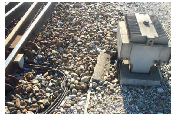
Resistor Transformer (old generation)
